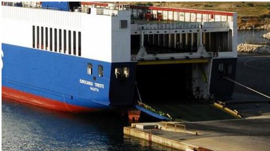
Figure 2: The single loading stern hydraulically driven ramp fitted on no. 2 garage deck (main deck).
